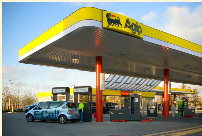
Hydrogen dispensers at the Agip service station in Frankfurt
